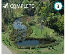
Wetland system filters surface runoff, protecting local wetlands and lakes.
