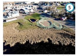
Stormwater treatment chain includes bioretention basins and an ironenhanced sand filter for water quality. Grants \$336,187
