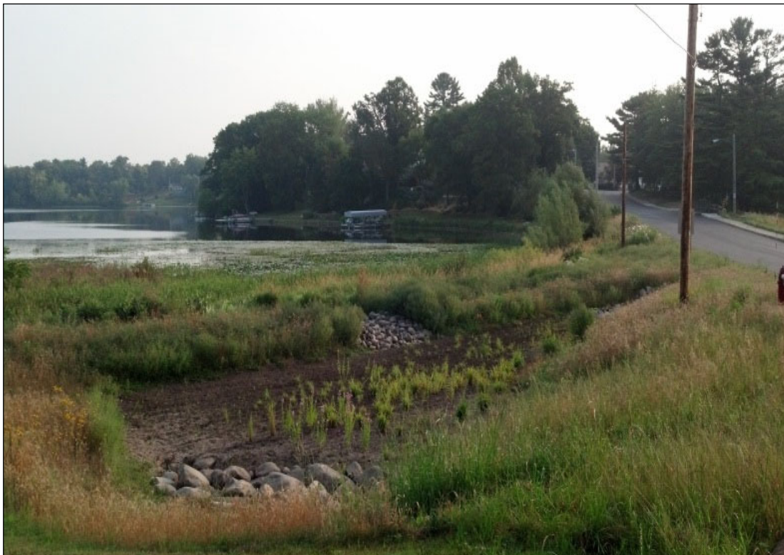
Stormwater runoff is treated by stormwater treatment ponds, including the stormwater treatment pond pictured above, before entering Library Lake. Photo Credit: EOR, Inc.
